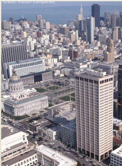
Aerial of 150 Van Ness Ave and Civic Center District Credit: Patson Companies
